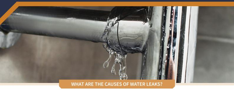
From a building / property perspective the causes of water leaks can include frozen pipes, taps being left on, poor quality pipe fittings, valve failures such as stopcocks, leaking appliances, overflowing sinks, blocked pipes, corroded pipework, and poor-quality installation.
